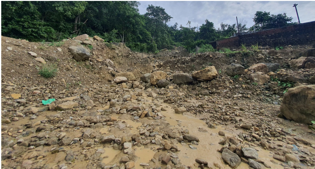
Figure 5: Debris flow in the existing water channel at the base of Shrrawan Danda (GPS: 27°42'44.71" and 83°28'15.44")
