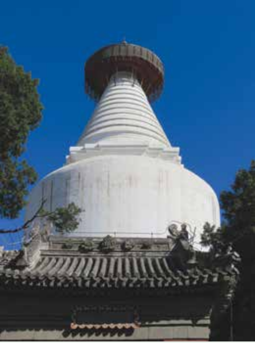
White stupa at Miaoying Temple, Beijing. Constructed by order of Kublai Khan under the supervision of Nepali architect Araniko, 1271.
