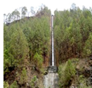
Figure 7: Steel Pipe of Kulekhani I at Jurikhet
