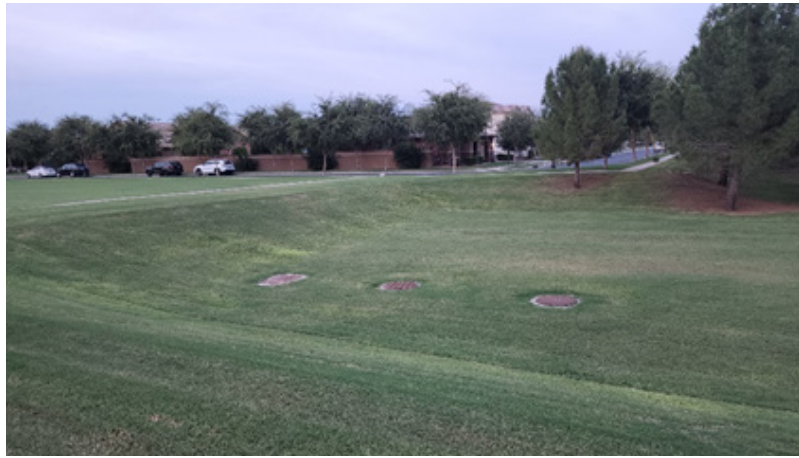
Figure 2. A retention pond in a residential development, Gilbert, AZ, USA. Photo by authors.
