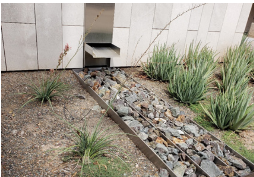
Figure 9. Redirecting rainwater to landscape irrigation in Tempe, AZ, USA. Photo by the authors.
