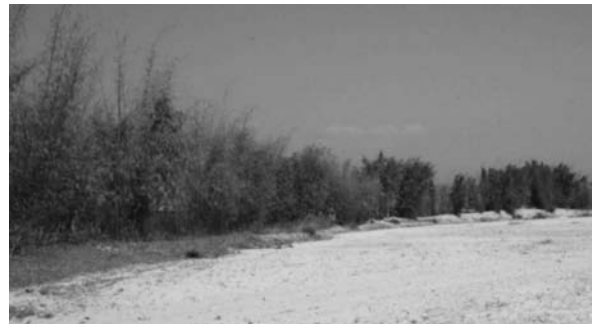
Photo 1 Bamboo wattle to stabilize slope and erosion control
