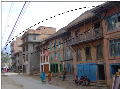
Fig 9 (b) Changing skyline in street facade
