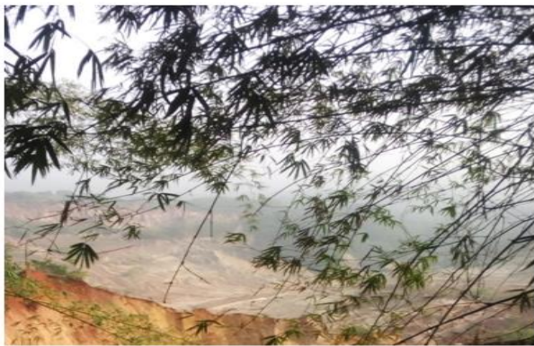
Plate 1: Humongous distortion of the landscape and destruction of agricultural land by the Oko gully, Orumba North Local Government Area, Anambra State
