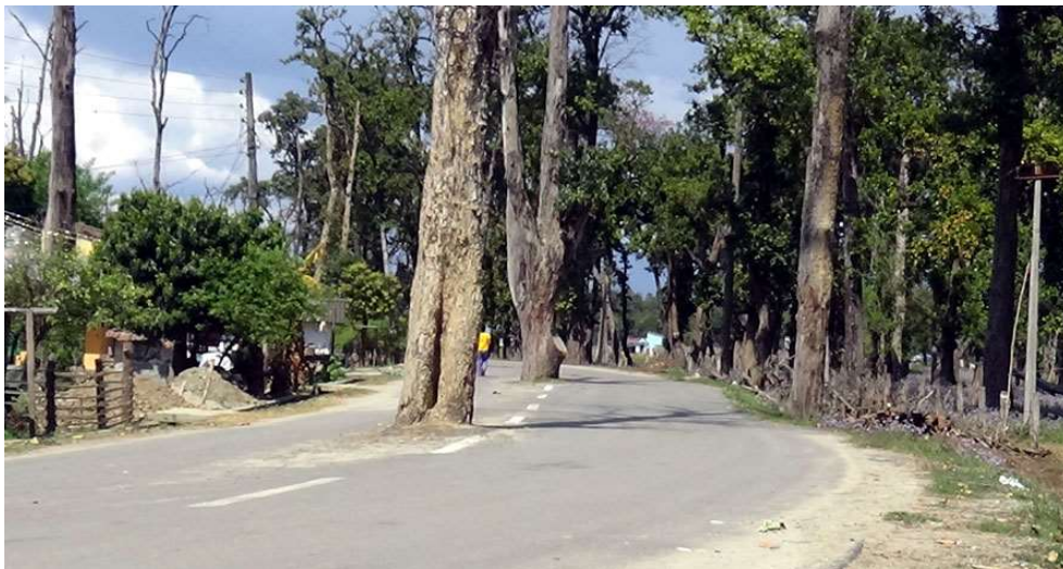
Figure 2: Road blacktopped in Dhangadhi without removing trees from the pavement (Bist, 2020)
