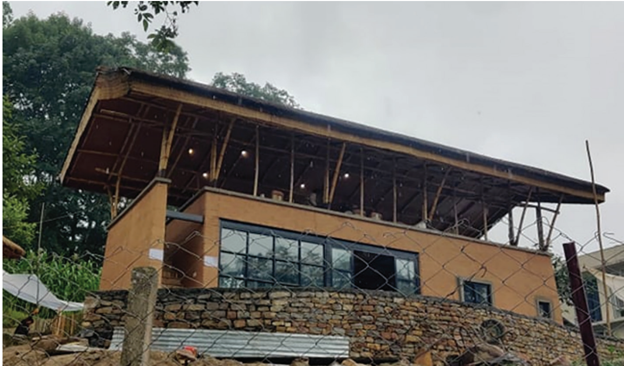
Figure 2: Case study building
