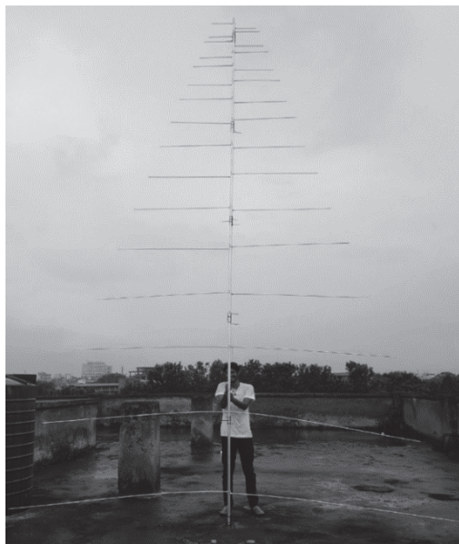
Figure 3: Fully fabricated antenna installed on Department of Electronics and Computer Engineering, Thapathali Campus, Kathmandu.
