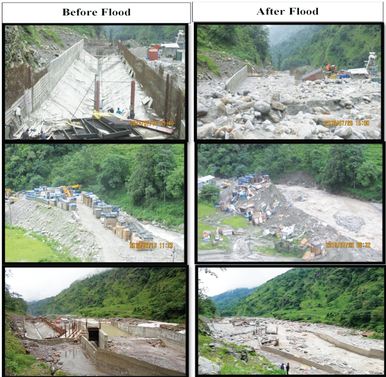
Figure 7: Comparative photographs of hydropower site before and after the flood.
