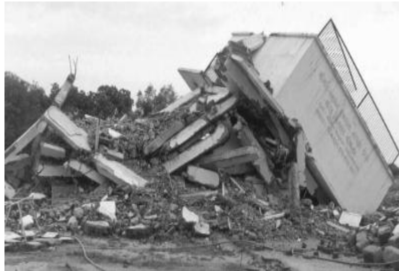
Figure 1: Collapsed Slender and Weak Framed Stagings of Water Tanks in Manfera Village [5]
