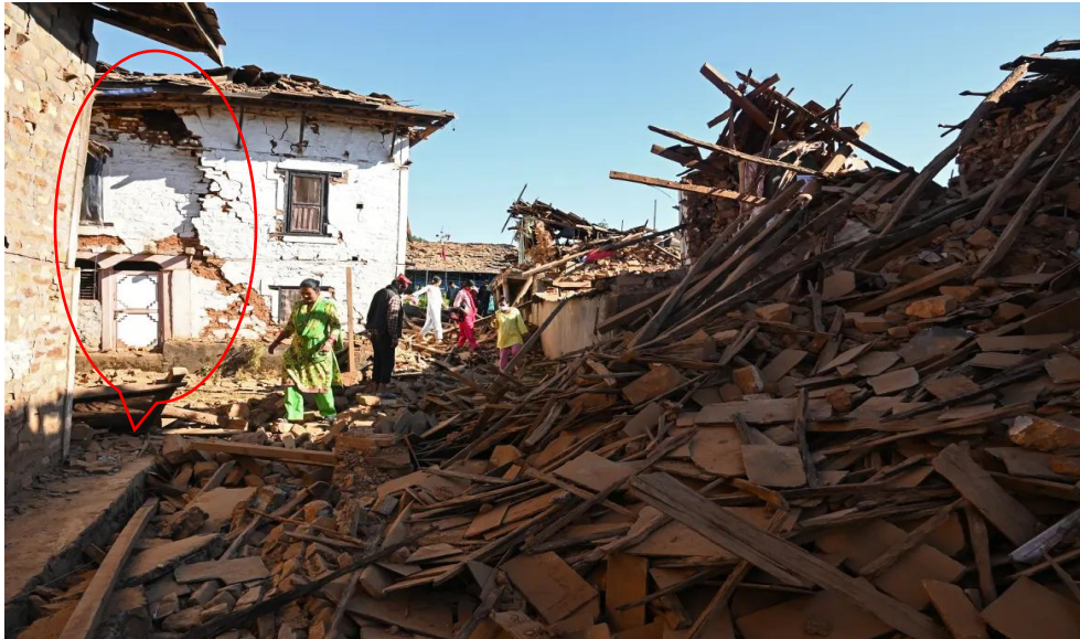
Figure 12: In-plane Failure of Exterior Walls
