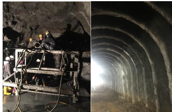
Figure 3: Excavation and Tunnel Support
