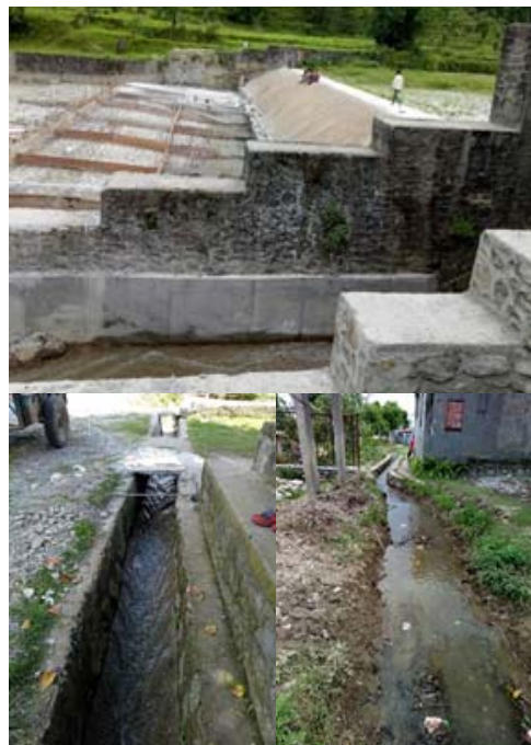
Figure 15: Headwork and canal at various reach of Hemja Irrigation System.
