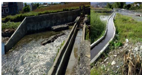
Figure 16: Headwork and main canal of Kimbesi Irrigation System
