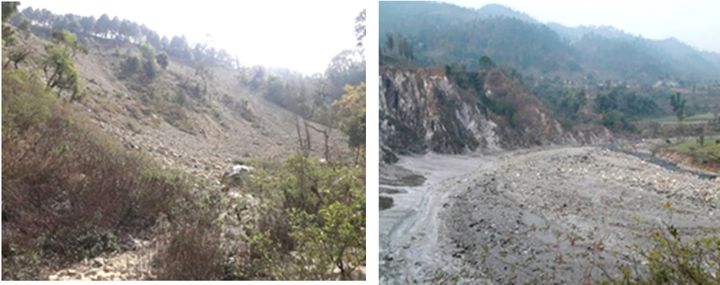
Photograph 3 and 4: Landslide of Sahajpur and Kimtola due to road construction and bank cutting of Thuligad
