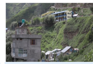
Photo 4.6: Private RCC Building and School building on the hillside (highway) (Shahi, Saroj)
