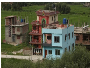
Photo 4.7: Private RCC Buildings with brick walls built on paddy field (Shahi, Saroj 2022)
