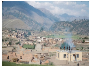
Photo 4.2: Stone Masonry Building under construction (Fairbank, 1971)
