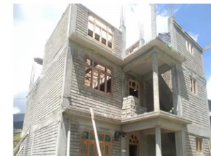
Photo 4.9: Building made of interlock brick locally made in Jumla (Magar, Amrit 2022)
