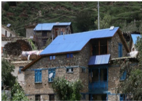
Photo 4.4: Stone Masonry Building with CGI Sheet Roof (Shahi, Saroj 2022)
