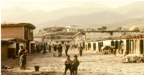
Photo 3.1: Main Market Area, Chandannath, Jumla (Fairbank, 1971)
