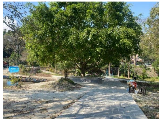
Figure 9: Newly constructed footpath
