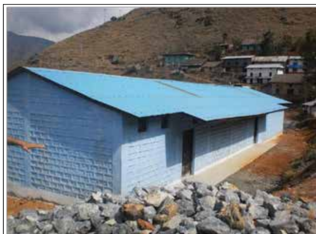
Newly constructed district medical stores in Rukum district
