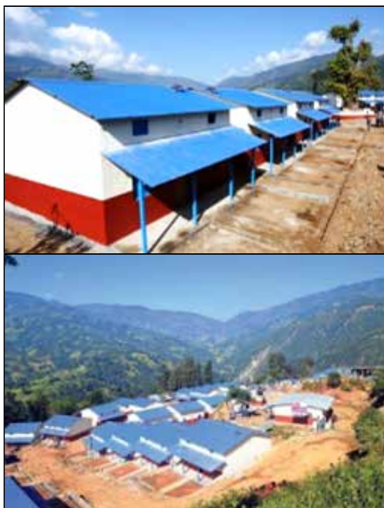
Photo 3: Houses of the Giranchaur integrated settlement for quake survivors, built by the Dhurmus Suntali Foundation, in Melamchi of Sindhupalchok district
