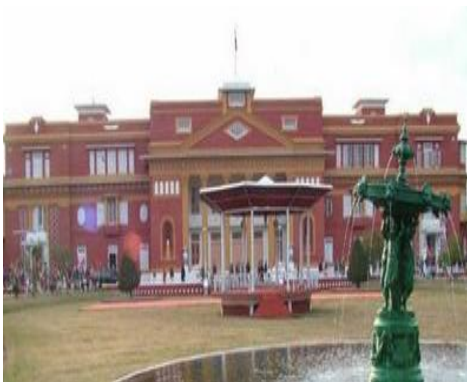
Figure 2 Present condition of Shital Nivas
