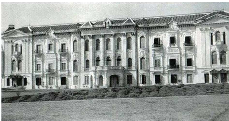
Figure 1 Shital Nivas before 1934 AD earthquake
