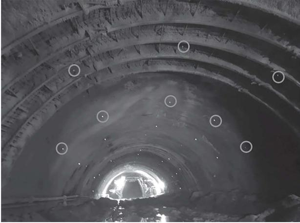
Figure 14: Optical Targets for Convergence Monitoring of the Tunnel
