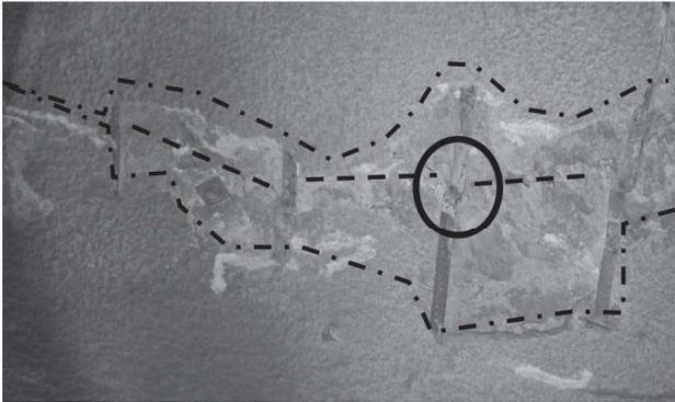
**Figure 6: Shotcrete spalling (dotted area in red) and steel rib twisting (red circle) along the longitudinal crack (blue dotted line)**
