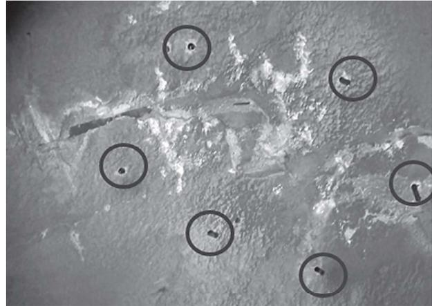
Figure 10: Grouting with hollow perforated pipe along the crack
