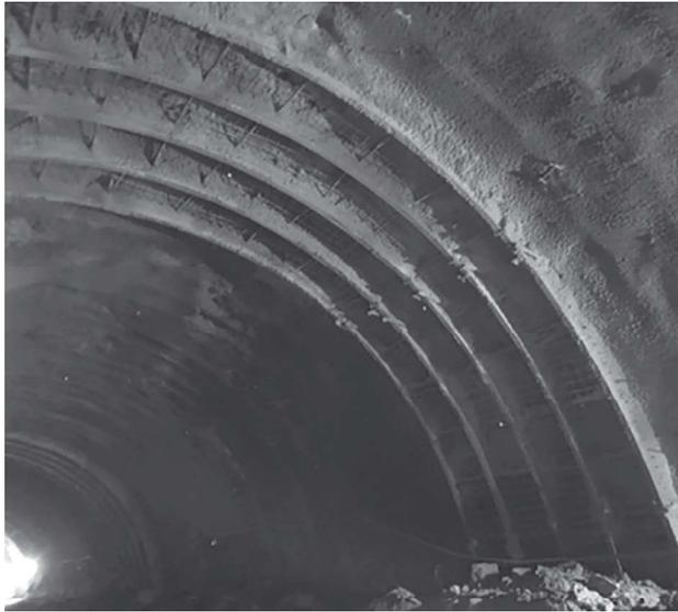
**Figure 13: Additional steel ribs installed inside the twisted steel ribs**
