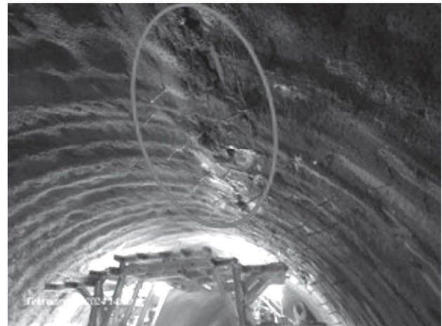
**Figure 9: deformation at right crown part**
