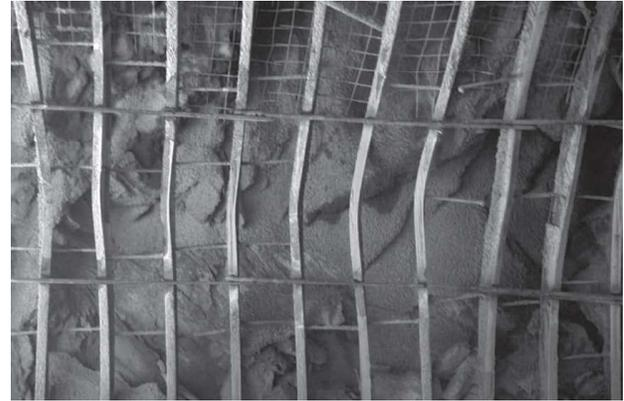
**Figure 8: Buckling of steel ribs without shotcrete**
