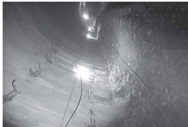
Figure 11: Foot locks for the steel ribs strengthening
