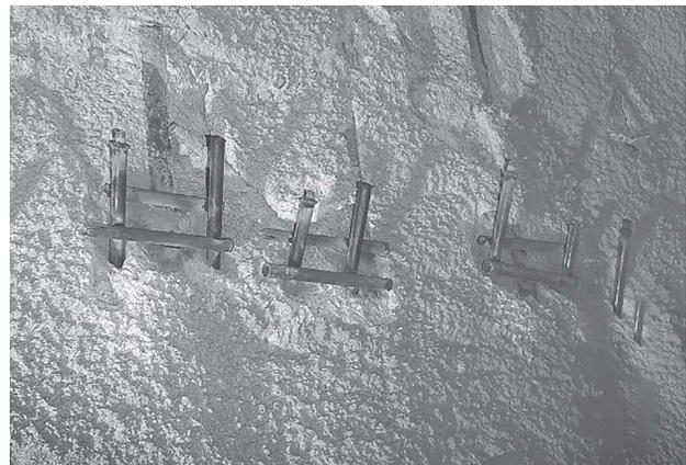
Figure 12: Foot locks for the steel ribs strengthening- a close view
