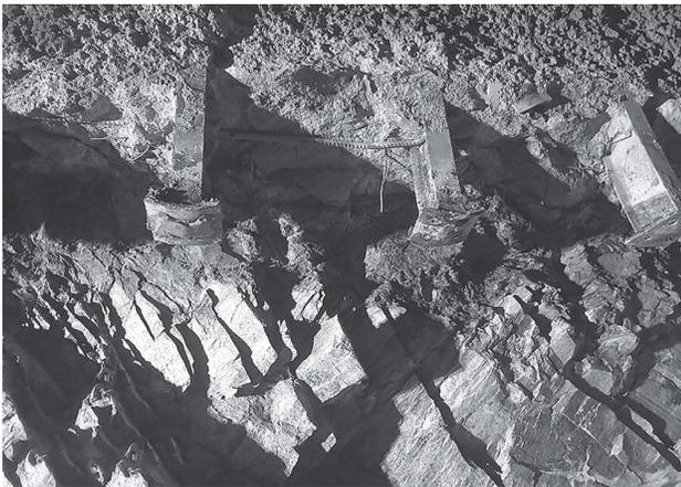
**Figure 7: Foot plate of steel rib heading part found punched while excavation of bench**
