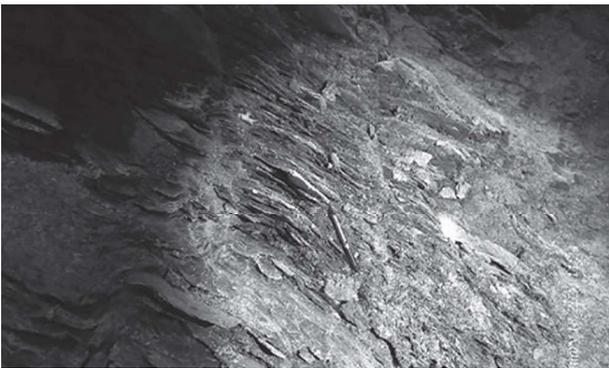
**Figure 4: Phyllite Rock mass exposed after excavation**
