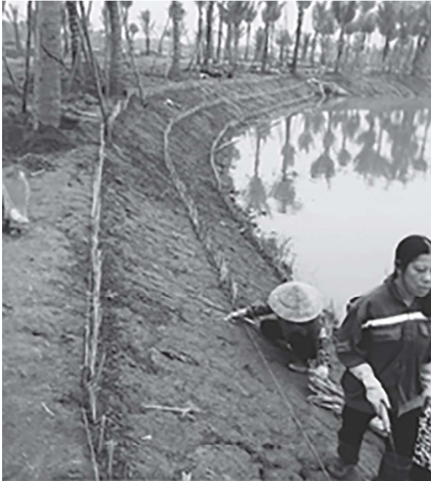
Figure 4: Riverbank stabilization in Vietnam
