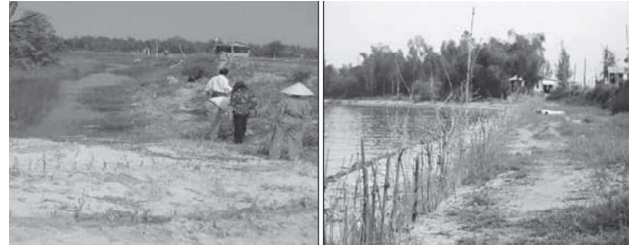
Figure 1: Left: March 2002: VS trial at the edge of a shrimp pond, where a canal drains flood water to Vinh Dien River; right: November 2002: mass planting combined with rock riprap to protect bank along Vinh Dien river.
