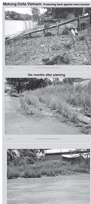
Figure 10: MEKONG DELTA VIETNAM: protecting bank against wave erosion
