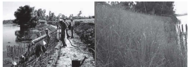
Figure 7: Left: Community members plant vetiver; right: November 2005: bank remains intact following the flood season
