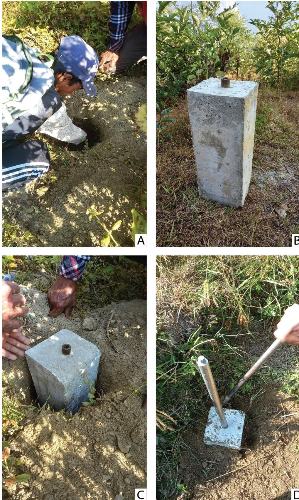
**Fig. 4:** Photographs showing the monumentation process, including A) digging the hole, B) concrete pillar installation, C) inserting the pillar, and D) rod setup for GPS device.
