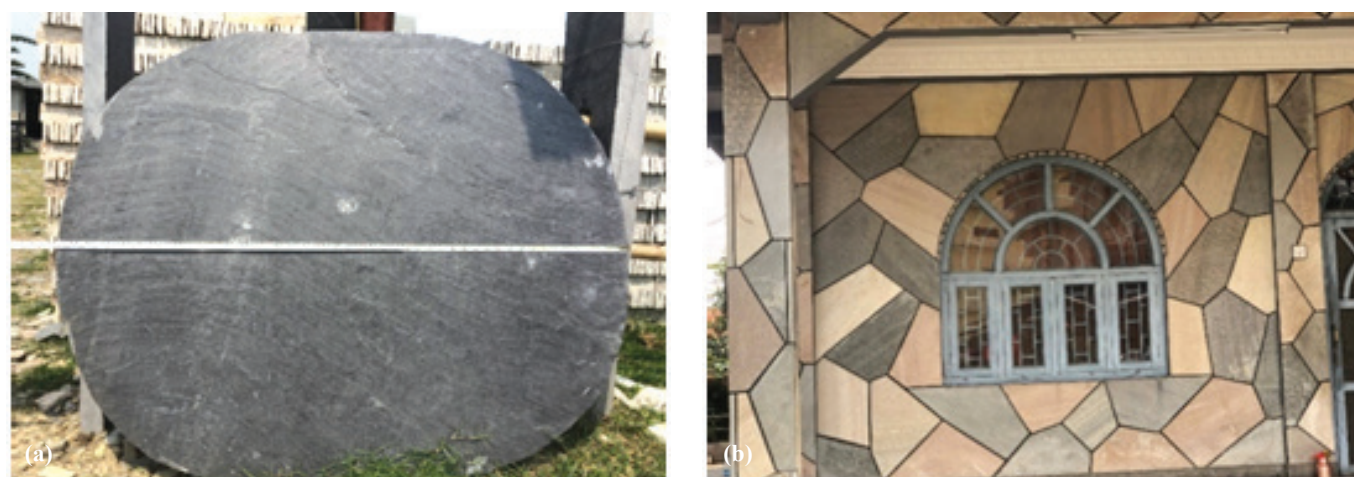
Fig. 2: The use of slate and quartzite as a dimension stone/cladding material in Pokhara city. (a) Slate (6 x 5 sq. ft) from Tarakhola for sale at Pokhara deposit, (b) wall of the house at Pokhara, cladding by Bhujrunghola pink quartzite and Tarakhola slate.
