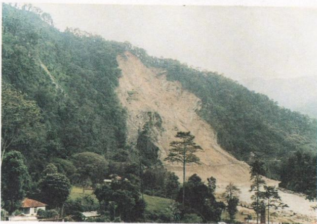
Plate 4: View of the Burdang Landslide by the Tista River
