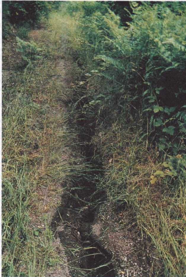
Plate 5: Failure along a track
