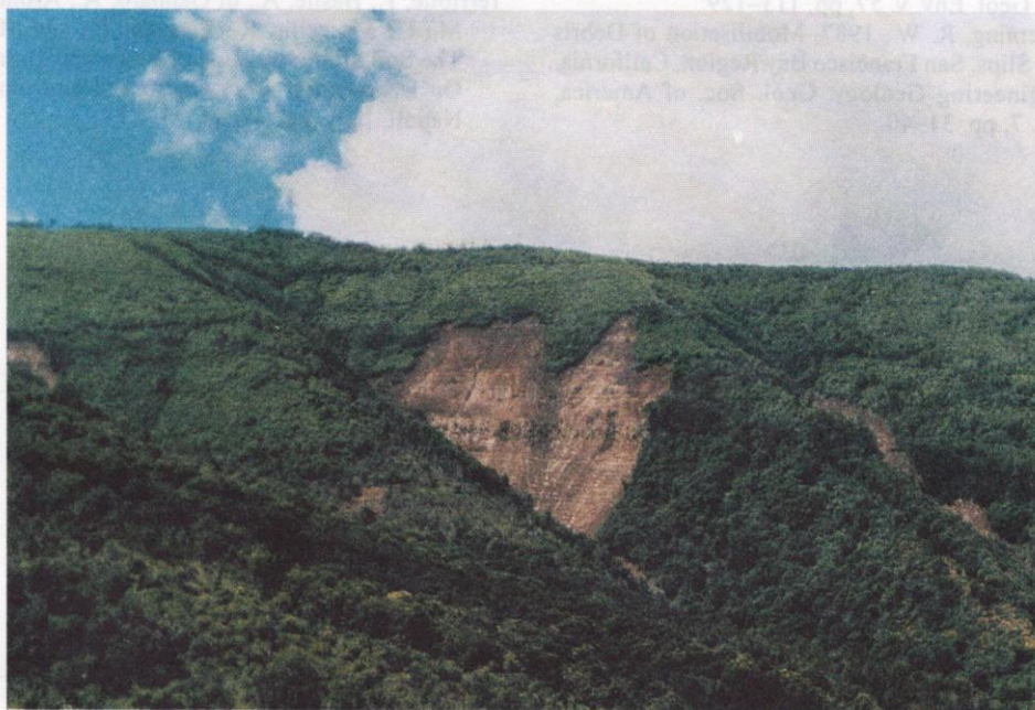
Plate 6: The shape of failure controlled by the geometry of track
