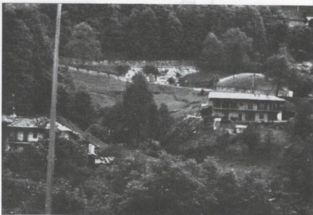
Plate 1: View of the landslide at Luserna, Italy
