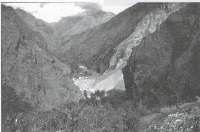
Plate 1: View of the village of Tatopani in the Kali Gandaki Valley upstream of the recent landslide, which has dammed the river to form a small lake along the village in the middle part of the picture. Note the steep joints in the quartzite member exposed in the left (western) foreground, and the relict failure scar on the right (eastern) front.
