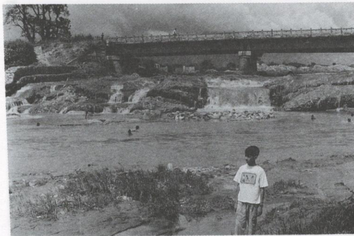
Plate 4: Failure of protection work and bridge, Manohara Bridge, Sanothimi in 1997
