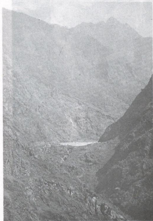
Fig. 3: The Lamabagar landslide dam (Dolakha district, eastern Nepal), showing a boulder armed spillway and a part of the entirely silted impoundment.
