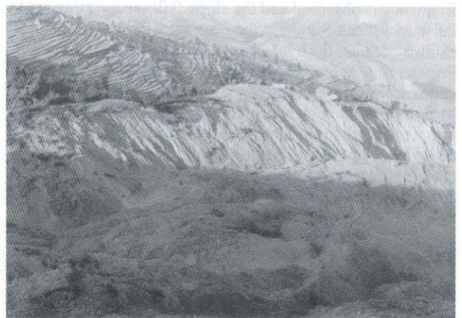
Fig. 9: Granular soil on a steep hill slope prone to failure
