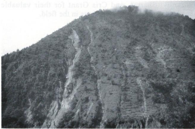
Fig. 17: A large erosive gully affecting four road levels. View to SW. Photo by Cris Grant.
