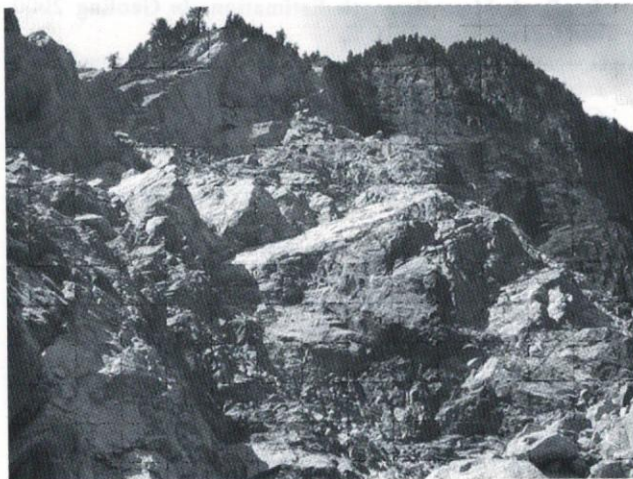
Fig. 10: Potentially unstable material in the failed zone
