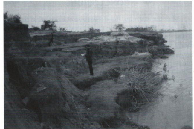
Fig. 9: Shear failure in the Brahmaputra River bank at Hatishal
