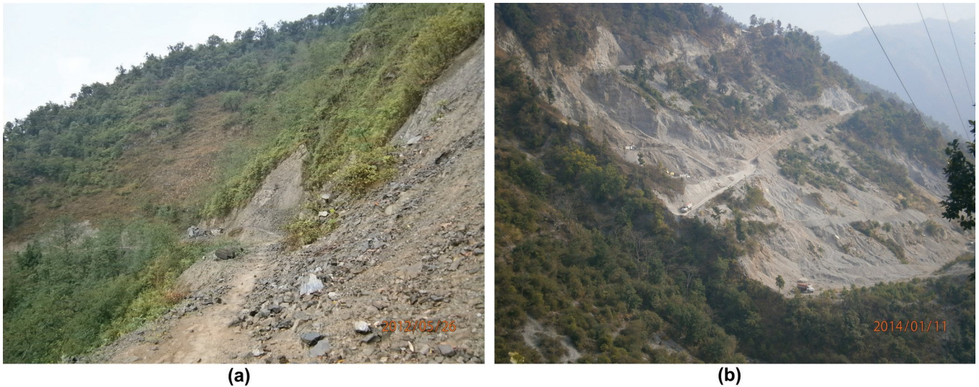
Fig. 7: Human intervention and landslide occurrences (a) road construction without due consideration of engineering geological conditions and (b) quarrying/mining activities.
