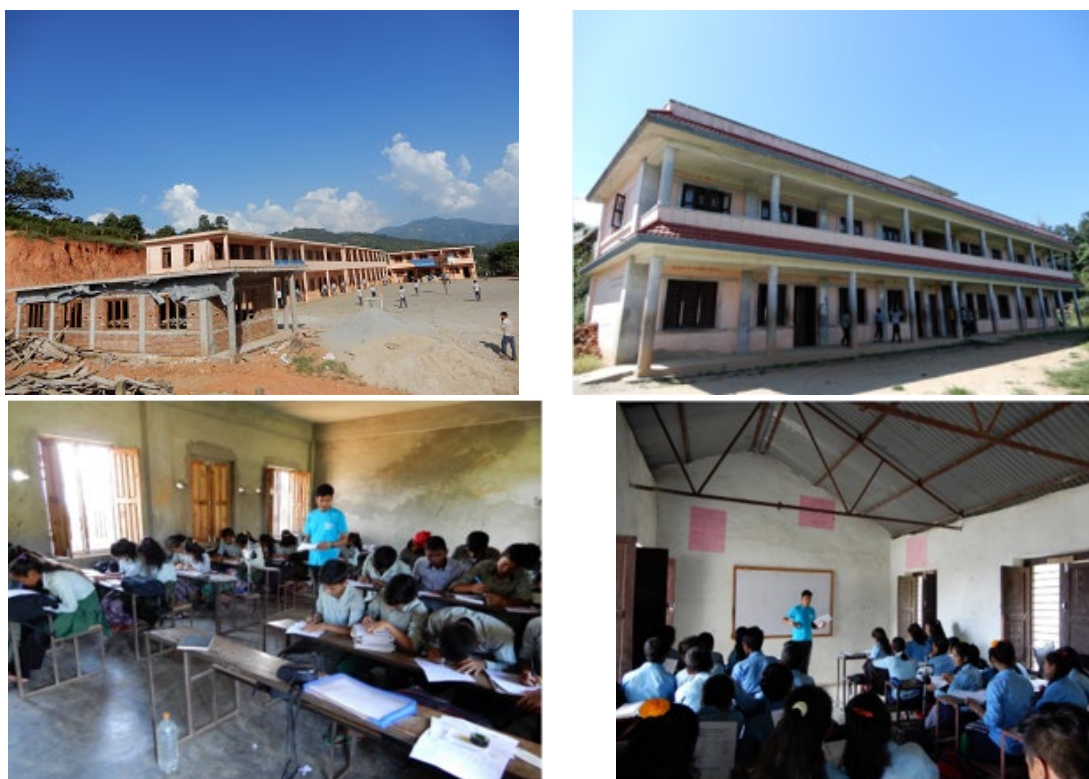
Figure 1: View of surveyed buildings and classrooms
