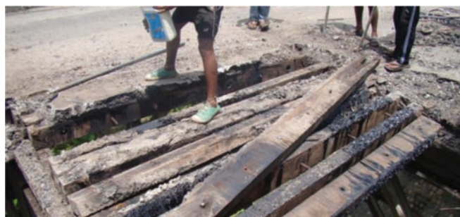
Fig. 3: Dismantling of Timber Deck
