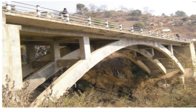
Fig. 1: View of Chobhar Arch Bridge
