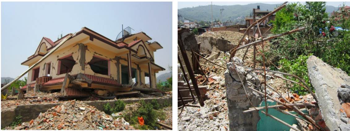
Figure 1. Collapsed RC frame building in Ramkot VDC, Kathmandu (left) and Close up view of its damaged exterior column (Right)
