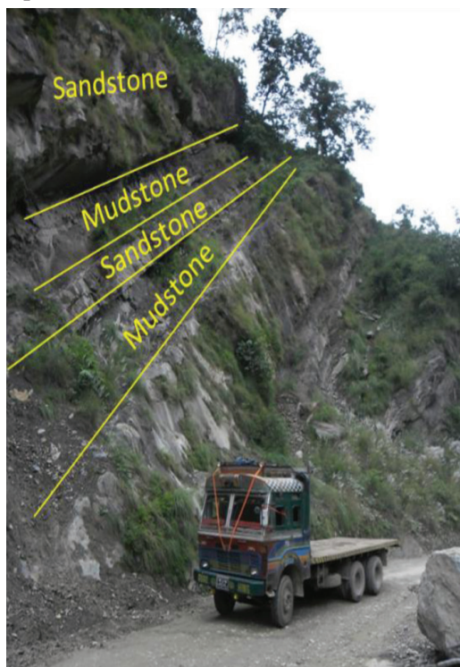
Fig. 4. The primary bedding is of sandstone and mudstone occurs at places; the mudstone bed erodes/wash out by rain then the overlying jointed rock loses support thus slips by plane failure
