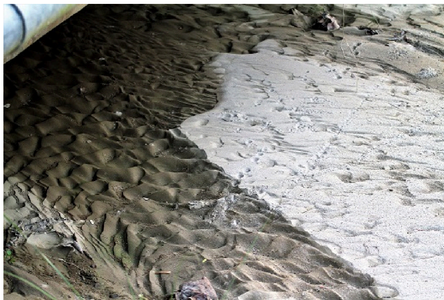
Fig. 4 Siltation may cause improper work of drainage structures
