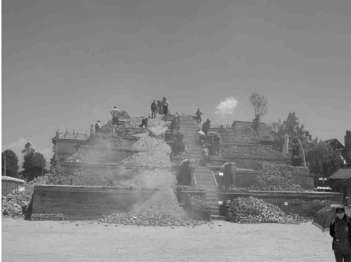
Figure 6: Fasi Dega Temple after Gorkha Earthquake 2015 (in cleaning stage) (Photo source: author)
