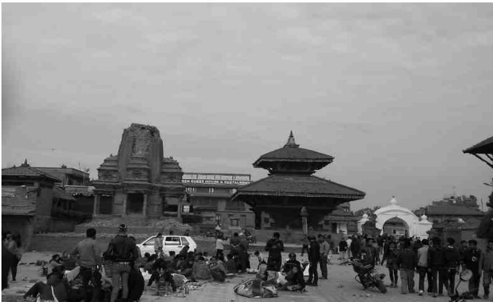
Figure 1: Damage of top part of Kedarnath Temple of Bhaktapur Durbar Square
