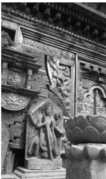
Figure 11: Damage in Changu Narayan Temple (North -West corner,bottom)
