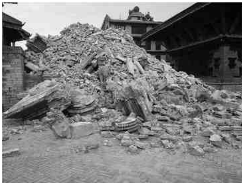
Figure 8: Collapse of Vatsala Durga Temple, Bhaktapur Durbar Square (Source: researchgate.net)
