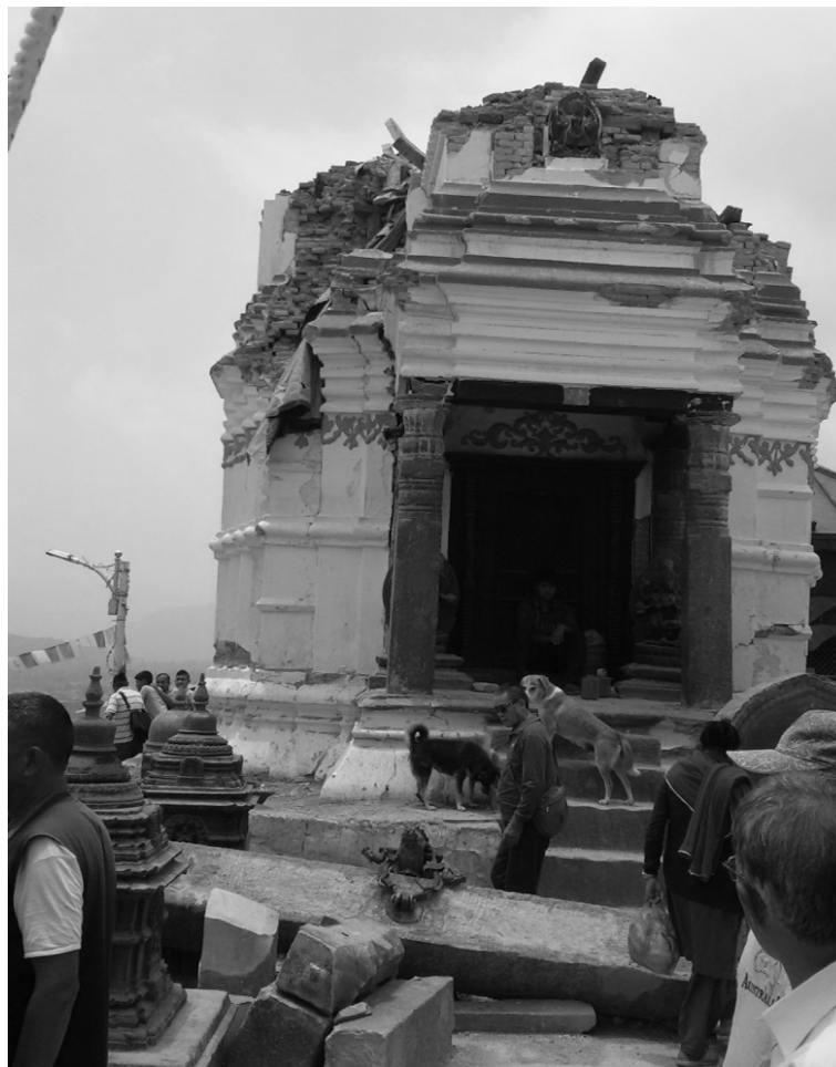
Figure 16 : Collapse of Anantapur temple in Swayambhu premises, Kathmandu
