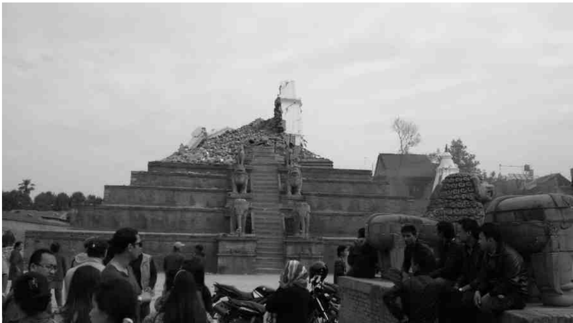
Figure 5: Fasi Dega Temple collapsed up to elevated top plinth(Photo source: author)
