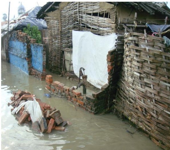
Figure 2. Impact of Flood on utilities.
