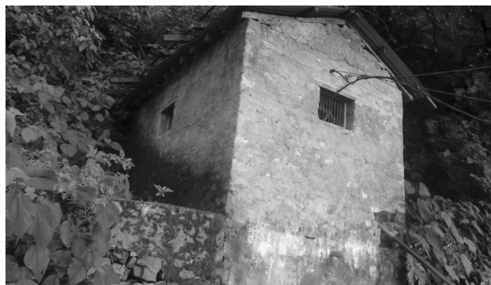
Photo 1. Intake of Water Source and Electric Panel Room
