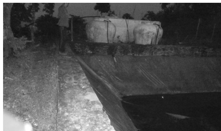
Photo 3. Water Collection Tanks for Drinking and Irrigation Purpose
