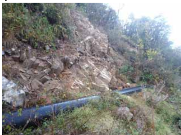
Photo1: HDP pipe functioning well in Earthquake triggered landslide
