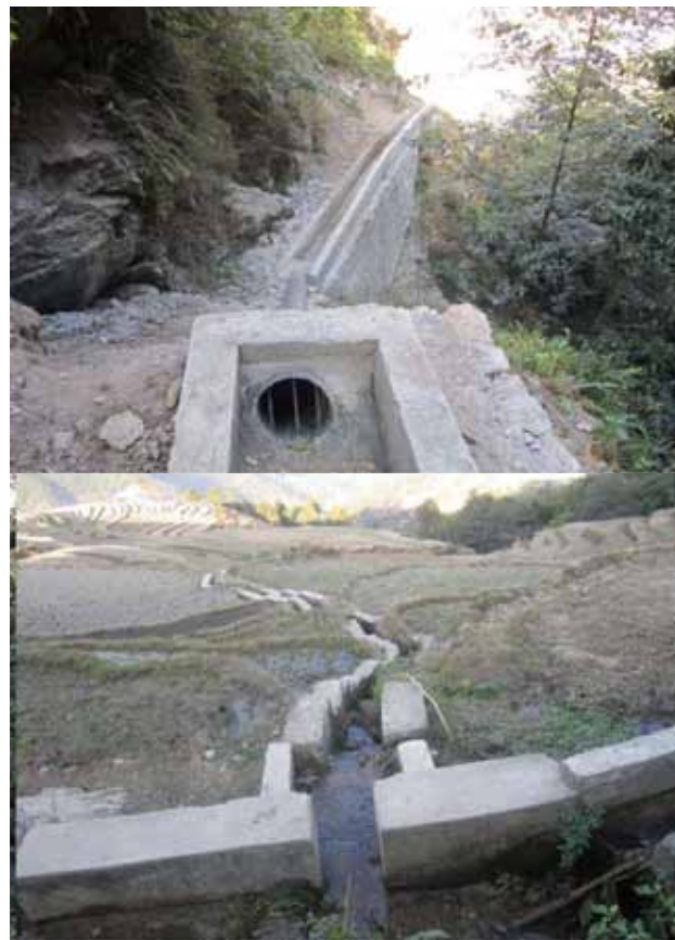
Photo 5: Comparison of pipe and masonry drops
