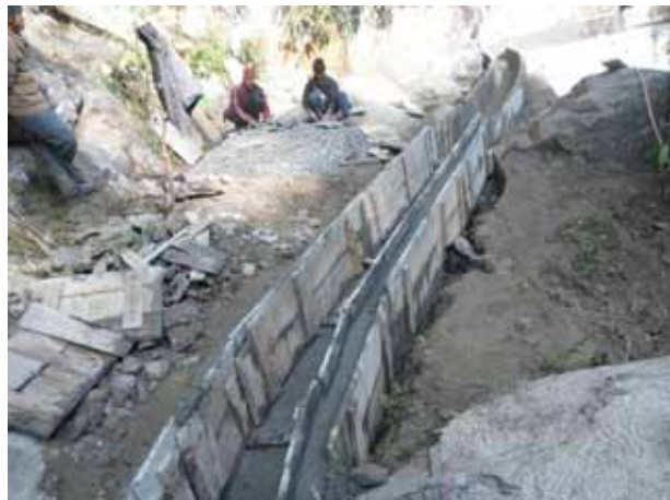
Photo 4: Cement concrete lining work includes a number of work steps
