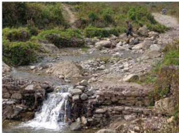
Photo 1: Old Canal Intake. (Photo courtesy: CIDD-5, Chitwan).
