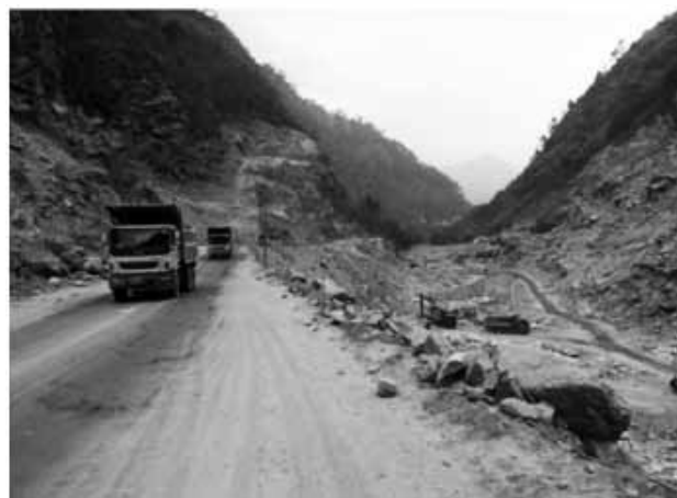
Photo 1. The ongoing Punatsangchhu construction in Punakha Wangdue valley
