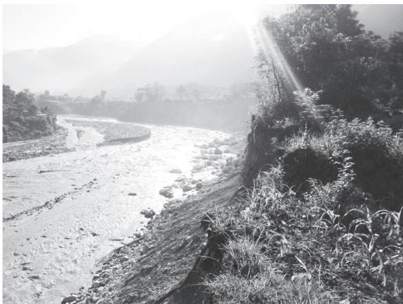
Figure 14. Deposition in India, Scouring in Nepal
