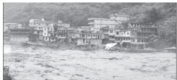
Figure 19. Attack by the flood on settlement
