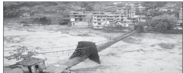
Figure 16. Nepal- India suspension bridge over Mahakali
