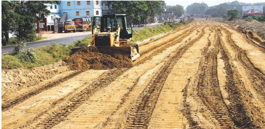
Fig. 5: Road construction near Dhaka, Bangladesh.
